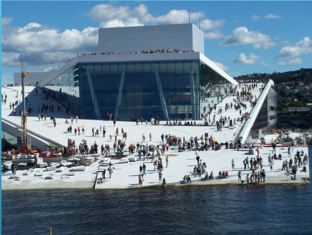
A. Oslo Opera House, Roof
